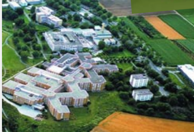
SLK-Hospital, Heilbronn realized by innovative Hospital Partner Imtech
