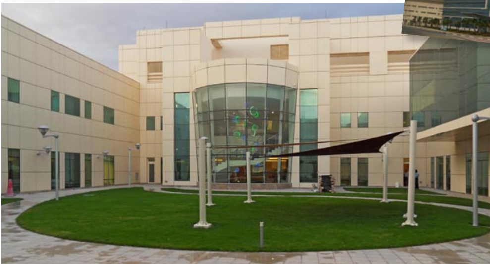
Dukhan Hospital, Qatar realized by innovative Hospital Partner Bender
